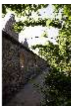
AschPomp.V, Laubengang (sog. Kapuzinergang), DI015031, BSV-
